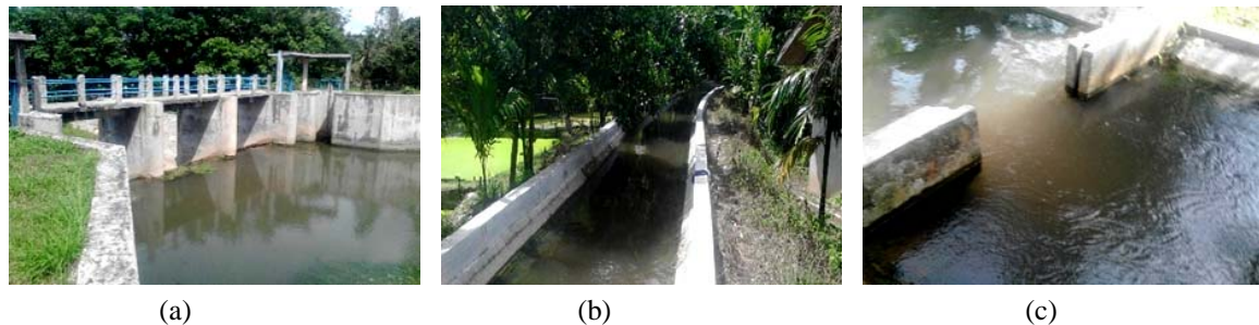
Fig. 1. The irrigation profile at Koto Tibun Village, (a) Small dam, (b) Irrigation channel, and (c) Spot testing
