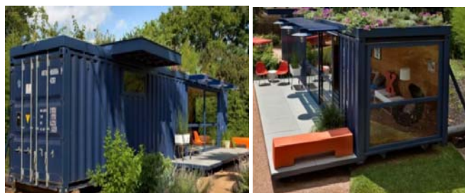
Fig. 16. Shipping container guest house by Poteet Architects. USA. 2010
