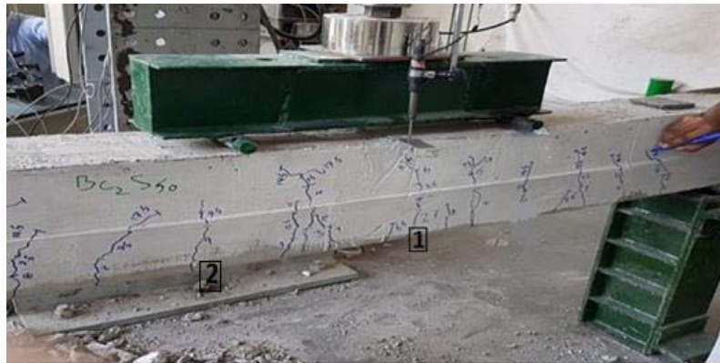
Figure2. GFRP reinforced beam
