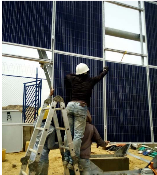
Fig. 5: Installation of solar panels
