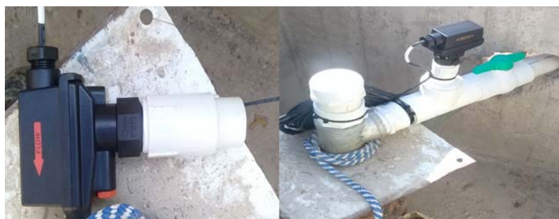
Fig. 10: Installation of sensors
