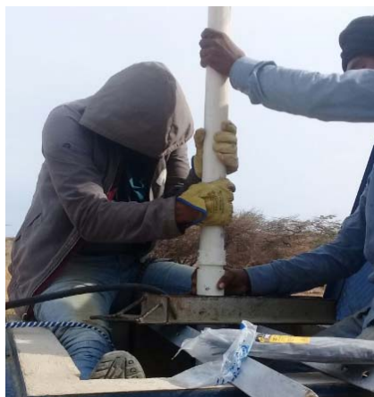
Fig. 9: Process of introduction of pump inside well
