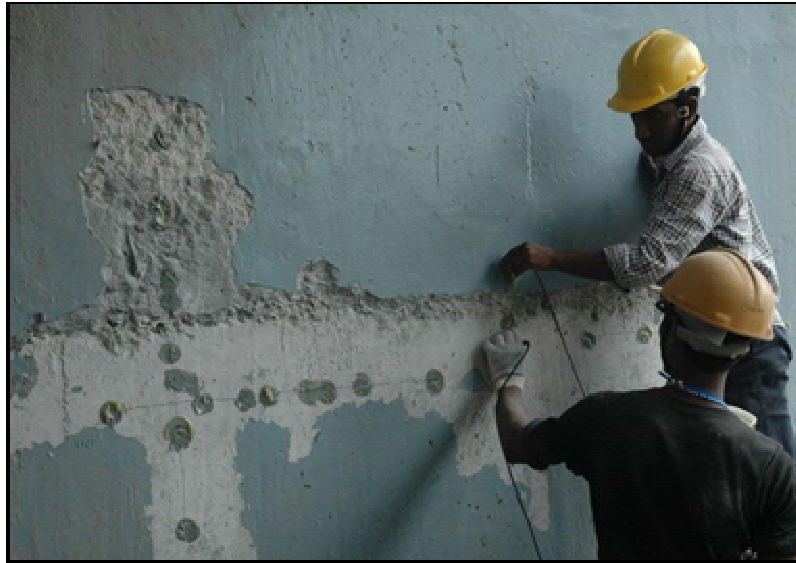
Fig.8: UPV testing is in progress.
