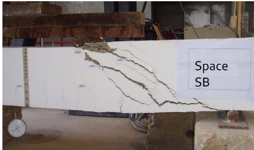
Fig. 7. Typical shear failure.
