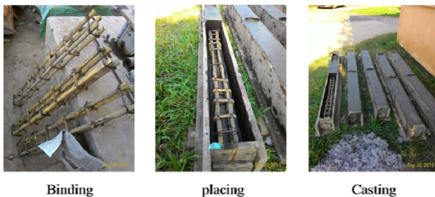
Fig. 6. Construction stages of bamboo reinforced beam.
