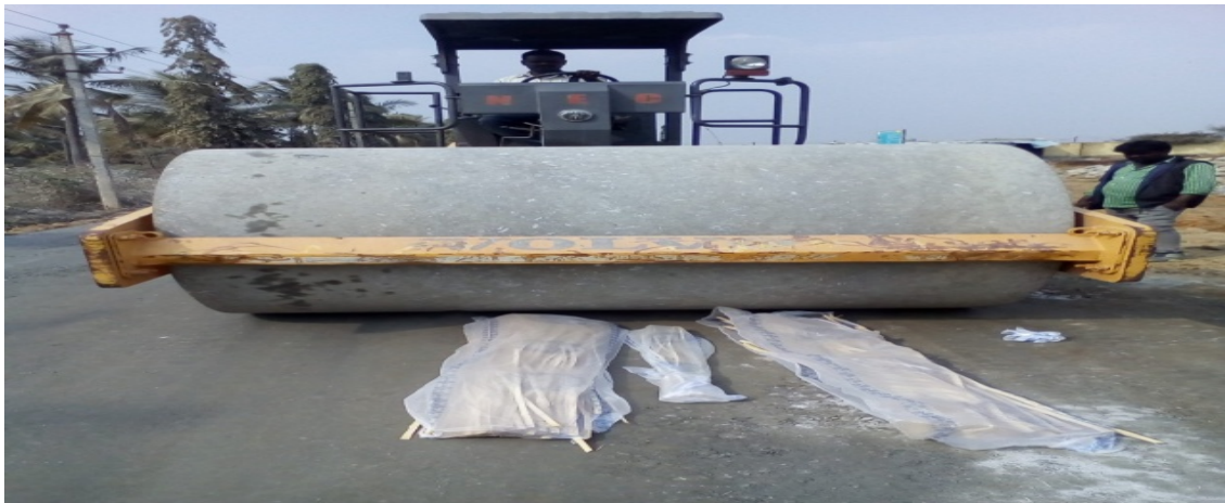
Fig. 4. Crushing of bamboo strips by roller
