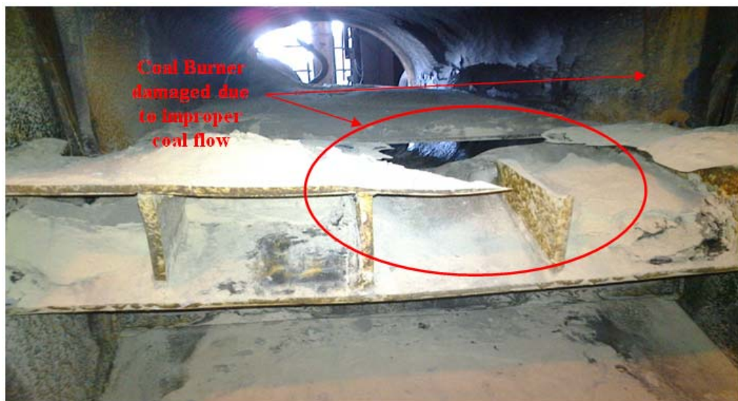
Fig. 2. Coal burner damaged due to improper coal flow.
