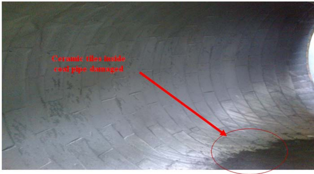
Fig. 1. Ceramic tiles damaged due to coal pipe de-choking work.
