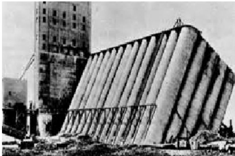
Fig.1.1. Illustration of the foundations's failure
