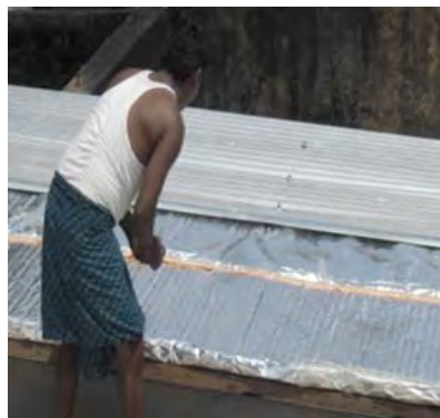
Fig.2 construction of DOD
