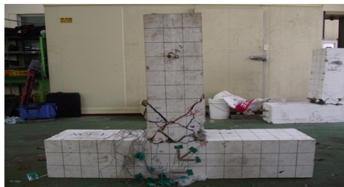
Fig.6. Fracture shape, NCJ-1
