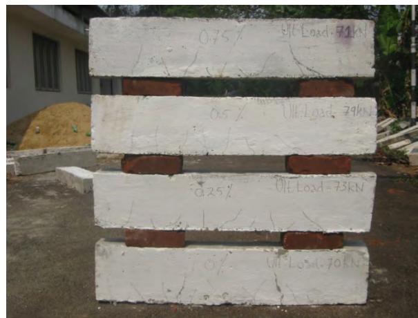
Fig. 14. Failure mode of M60 Beams- 3rd day
