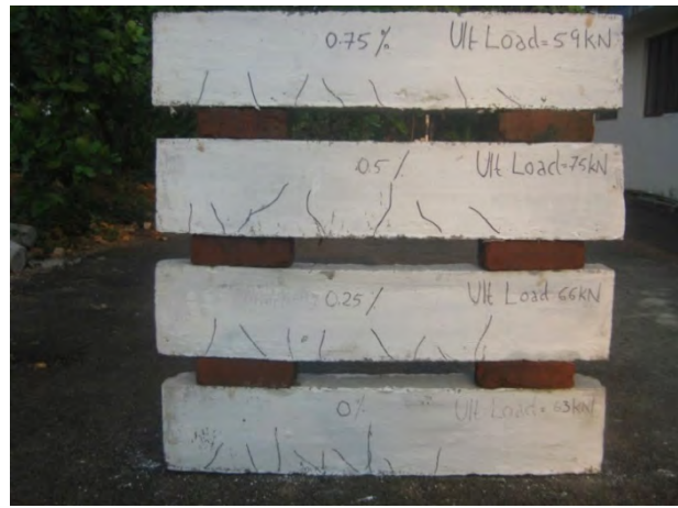
Fig. 11. Failure mode of M40 Beams- 3rd day
