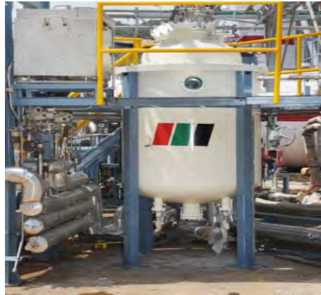
Fig. 4. Photograph of Super Insulated Dewar with fluid circuits
