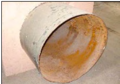
Fig. 3. Forsaken pipe due to a critical value of thickness
