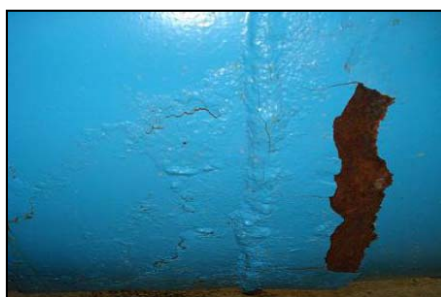
Fig. 11 – Corrosion under the paint frame
