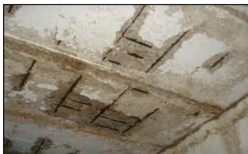
Fig. 5. State of the roof and walls affected by the humidity (Metal reinforcement is corroded)
