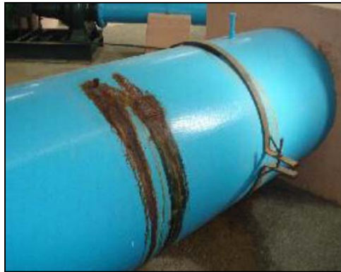
Fig. 2. Water leakage due to cracks; internal corrosion is suspected
