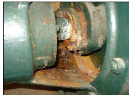
Fig. 4. – Corrosion on the drive shaft of a pump
