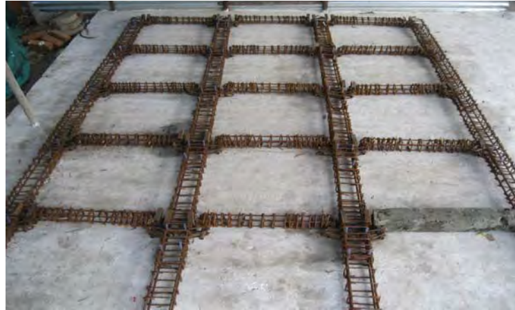
Fig. 2. Reinforcement for Prefabricated frame
