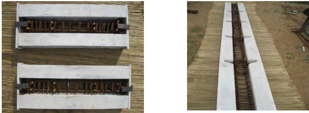
Fig. 3(a). Mould and reinforcements for preparation of precast beam and column specimens
