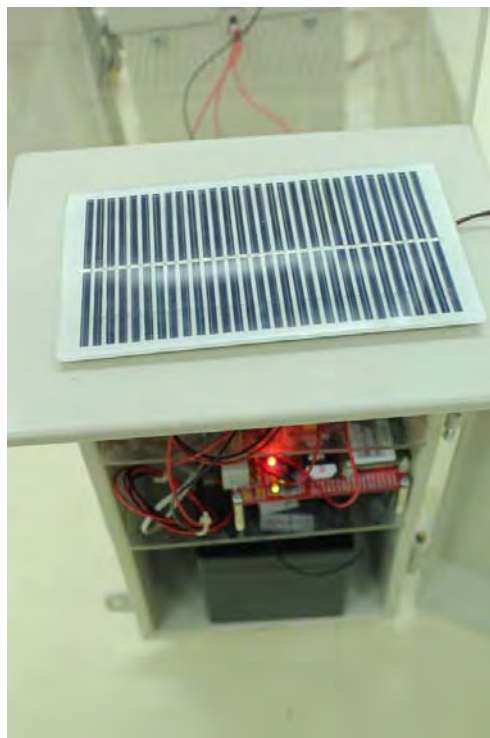
Fig. 7: The solar cell and control unit
