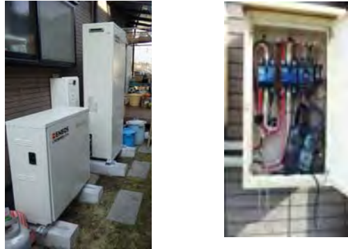
Fig.1 Appearance of a 1 kW PEFC system
