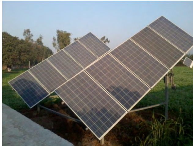
Figure 3: SPV based water pumping system at the Jasvinder Singh Farmhouse, Kota
