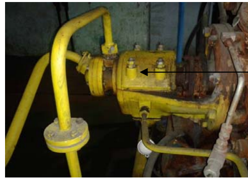
Figure n°8: bearing n° 4 pump side
